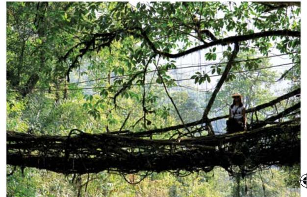
**ABOVE** Locals have ingeniously adapted the rubber trees *Ficus elastica* to create swaying root bridges that can withstand the incessant and heavy rains that bathe the region.
